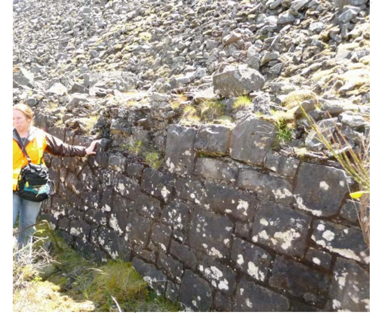
Historic masonry wall at Shellrock Mountain.
