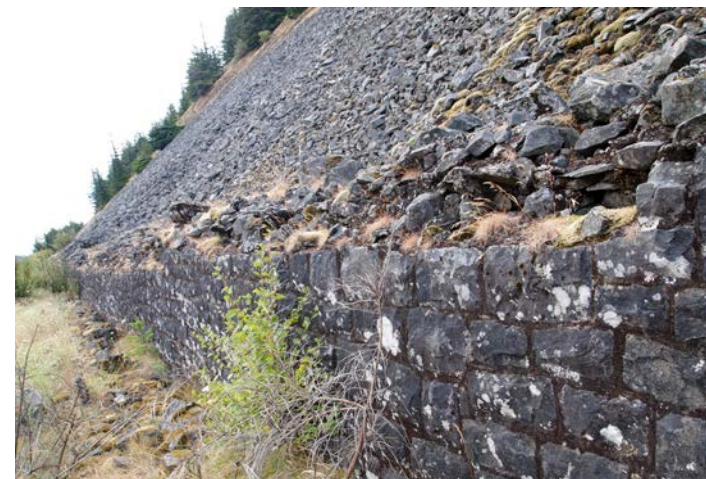
Historic masonry wall at Shellrock Mountain.
