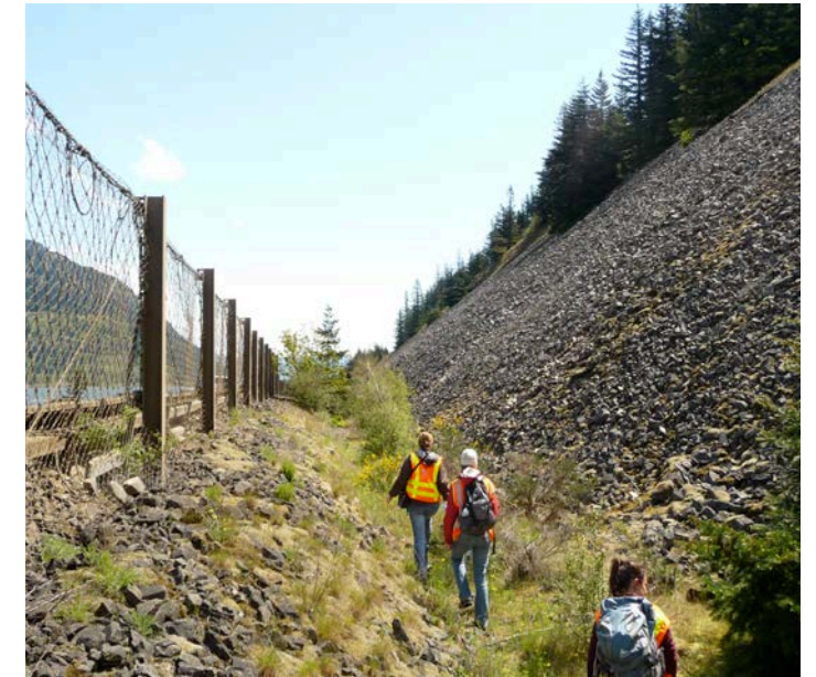
Existing condition behind bin wall.
