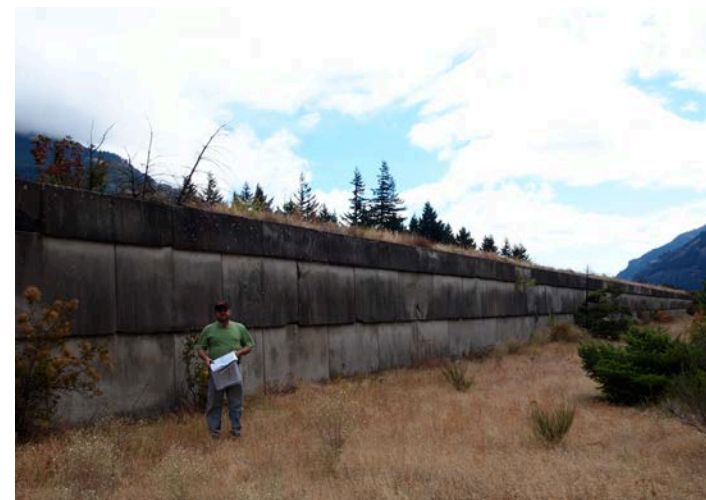
Existing concrete bin wall east of Summit Creek.
