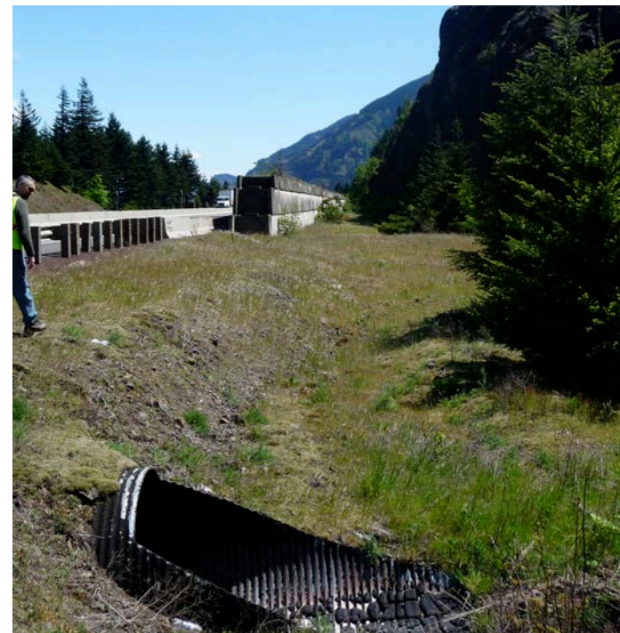
View of Summit Creek culvert west of bin wall.
