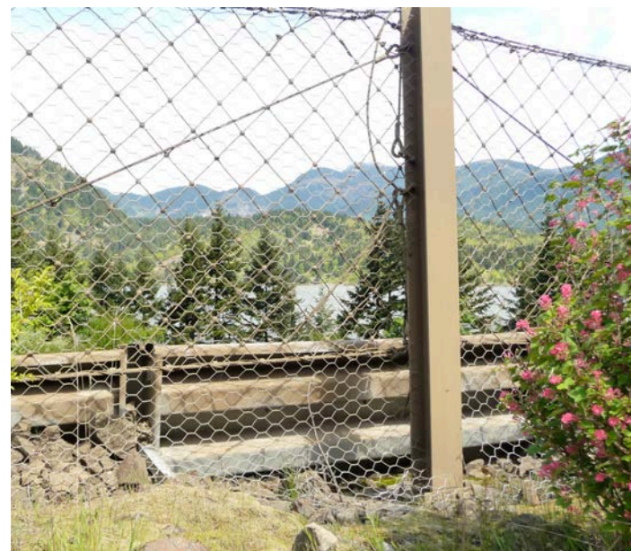
Existing rockfall fence and back of bin wall.
