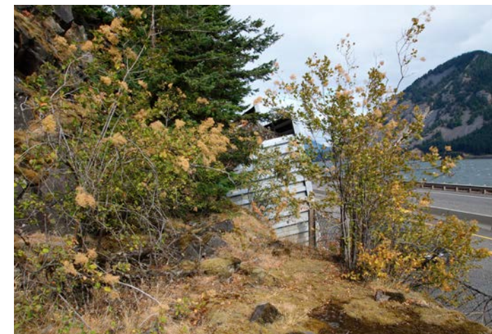
Existing section of Historic Highway at metal bin wall.
