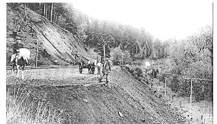
Construction of Highway at Lindsey.
