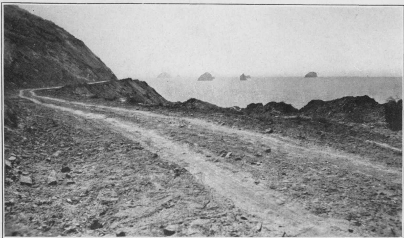
A NEWLY GRADED SECTION ON THE COAST HIGHWAY IN CURRY COUNTY.
