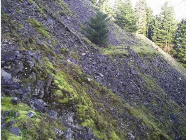
Figure 42. View of the rock-faced road showing dry-stacked cobble and boulder construction.
