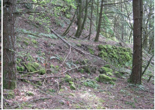
The rock-walled road segment west of the small creek crossing, view northwest.
