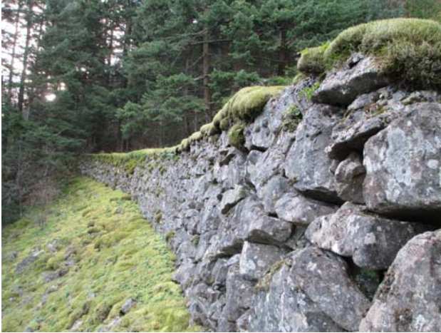
Figure 42. View of the rock-faced road showing dry-stacked cobble and boulder construction.
