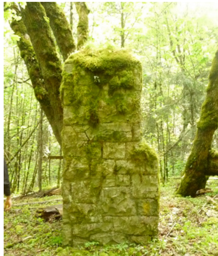
Existing masonry sign base at Perham Creek.
