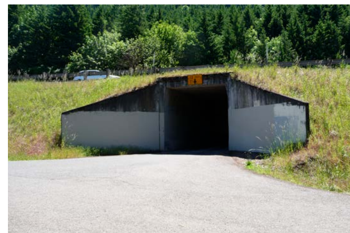
Existing tunnel under I-84.
