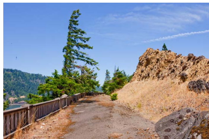
Existing Highway viaduct section at Ruthton Point.
