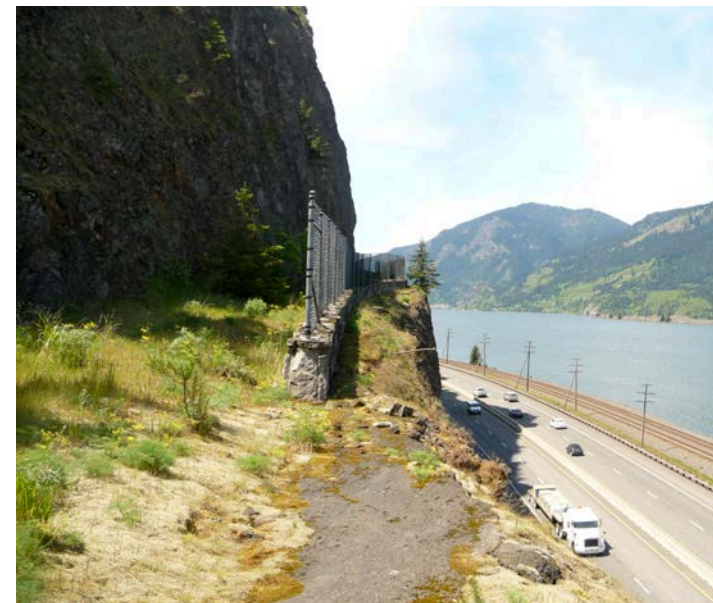
View looking toward location of historic tunnel at Mitchell Point.
