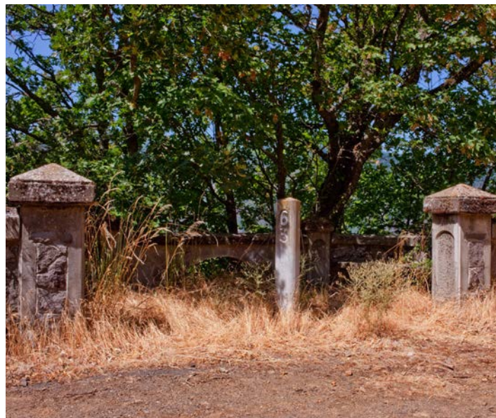
Restored Milepost 63 at Ruthton Point.
