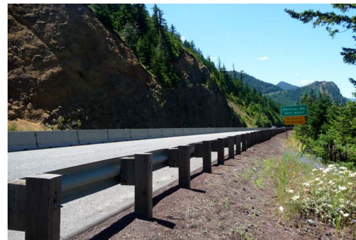
Existing conditions at I-84 west of Ruthton Point.
