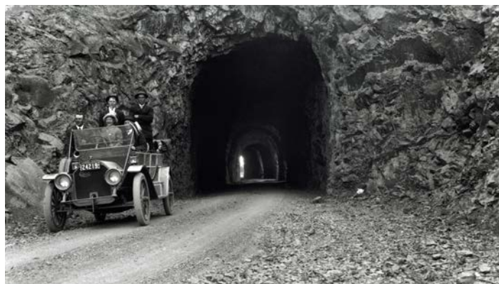
East side of Mitchell Point Tunnel.
