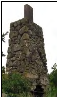
Figure 3.33: Crag Rats Club House Chimney
