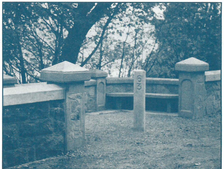
Transformed Ruthton Point.
