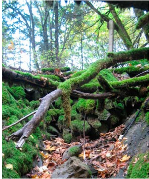
Detail, rubble headwall, Cabin Creek
