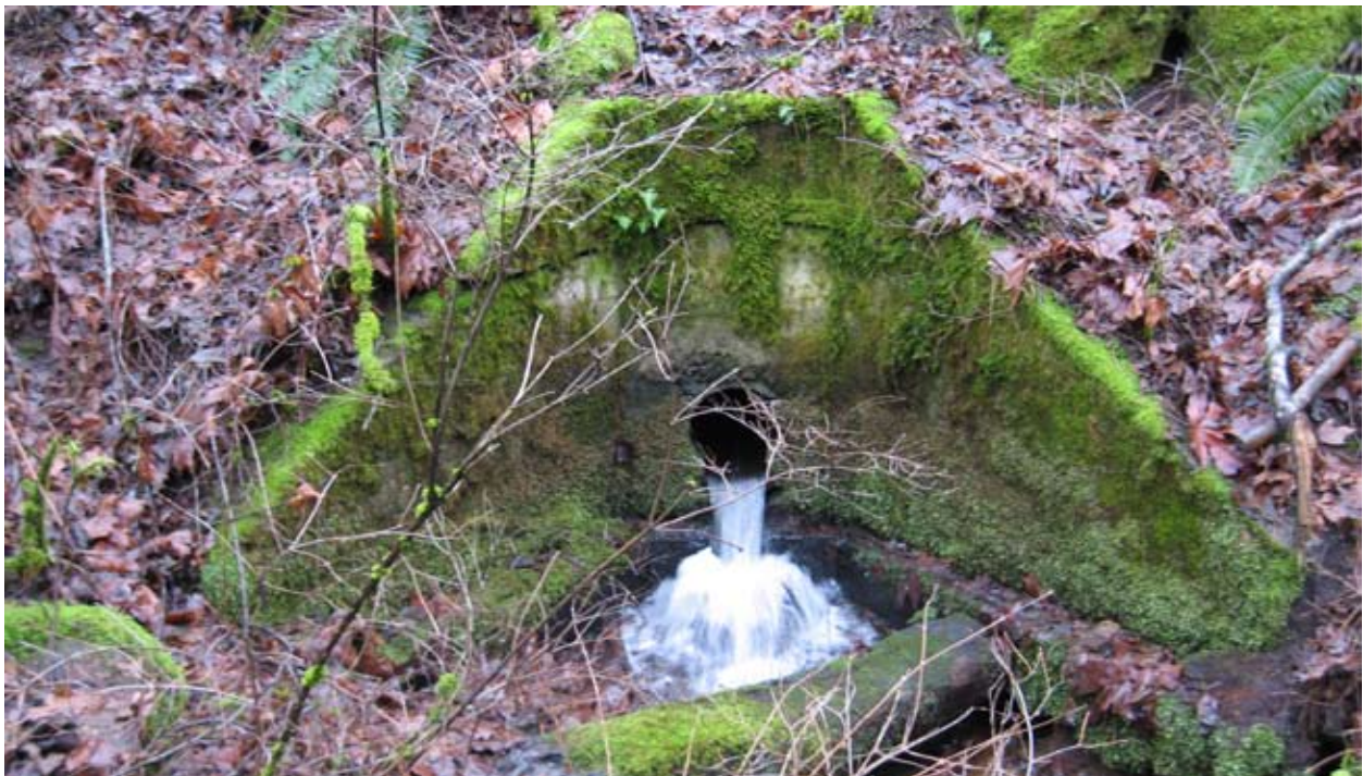
Concrete culvert headwall, Mitchell Point East.
