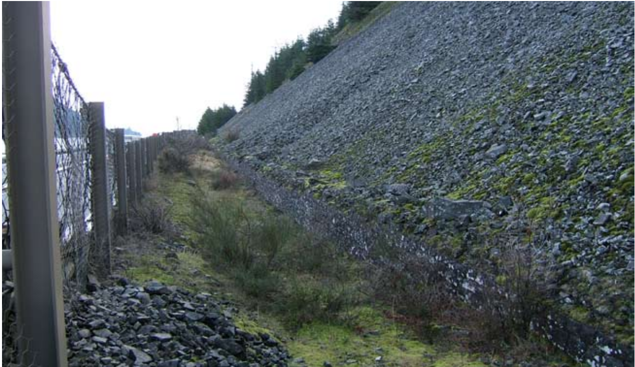
Retaining wall and rock catchment, Shellrock Mountain
