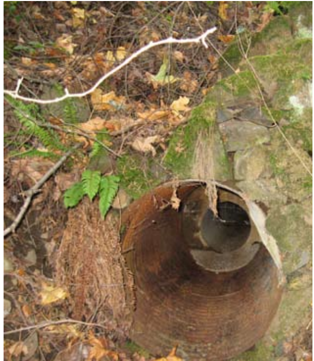
Culvert, rubble wall, Mitchell Point 2
