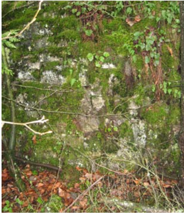
Retaining wall, Shellrock Mountain
