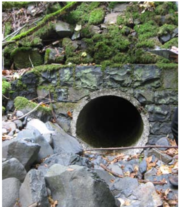
Cabin Creek culvert
