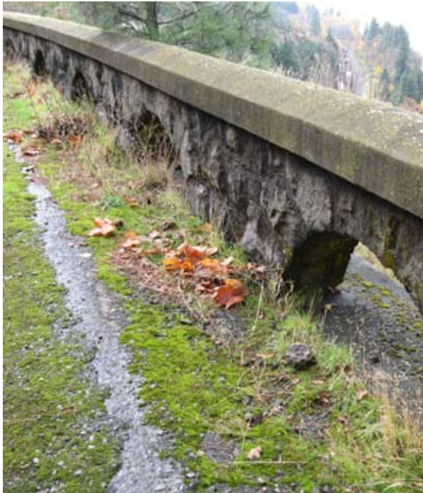
Restored Masonry Parapet, Ruthton Point
