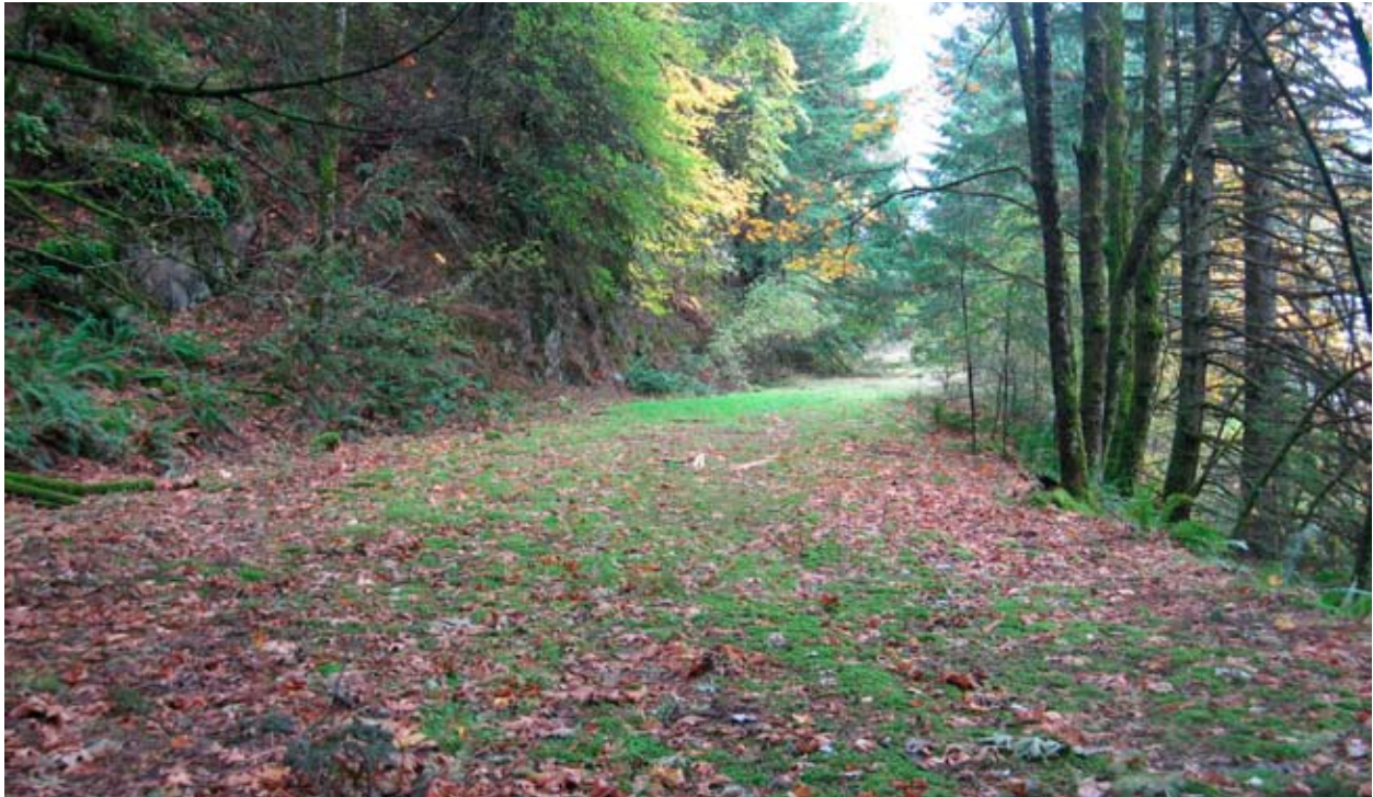
Road surface, alignment, rock cut. Lindsey Creek Segment.
