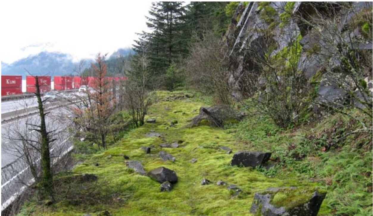
HCRH roadbed and rock cut, Shellrock Mountain
