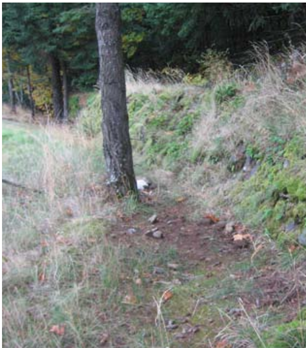
Retaining Wall, Cabin Creek Area
