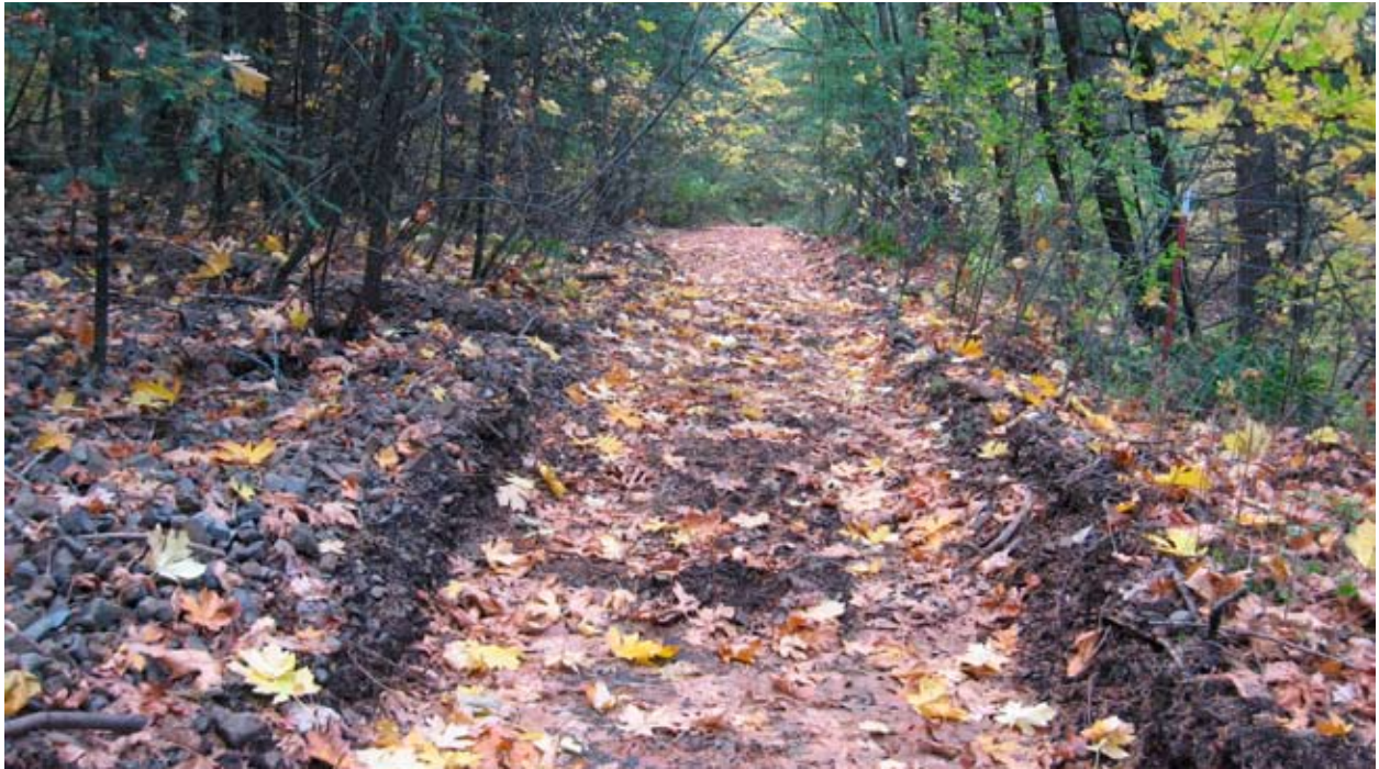
Washed out, buried road bed, Viento Segment 1. Contemporary wire fence on right.
