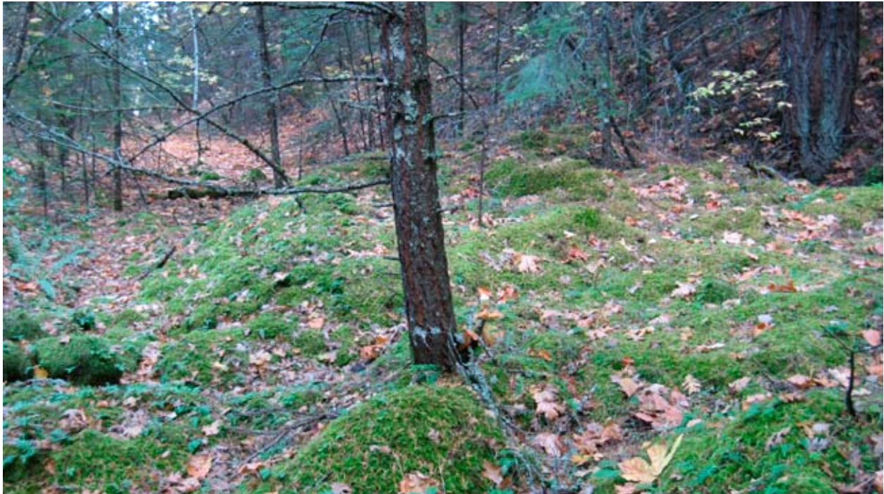
Pile of asphalt and rubble from removed roadbed, Viento Segment 3. The roadbed in the background has buried, fragmented pavement in poor condition, overgrown vegetation.
