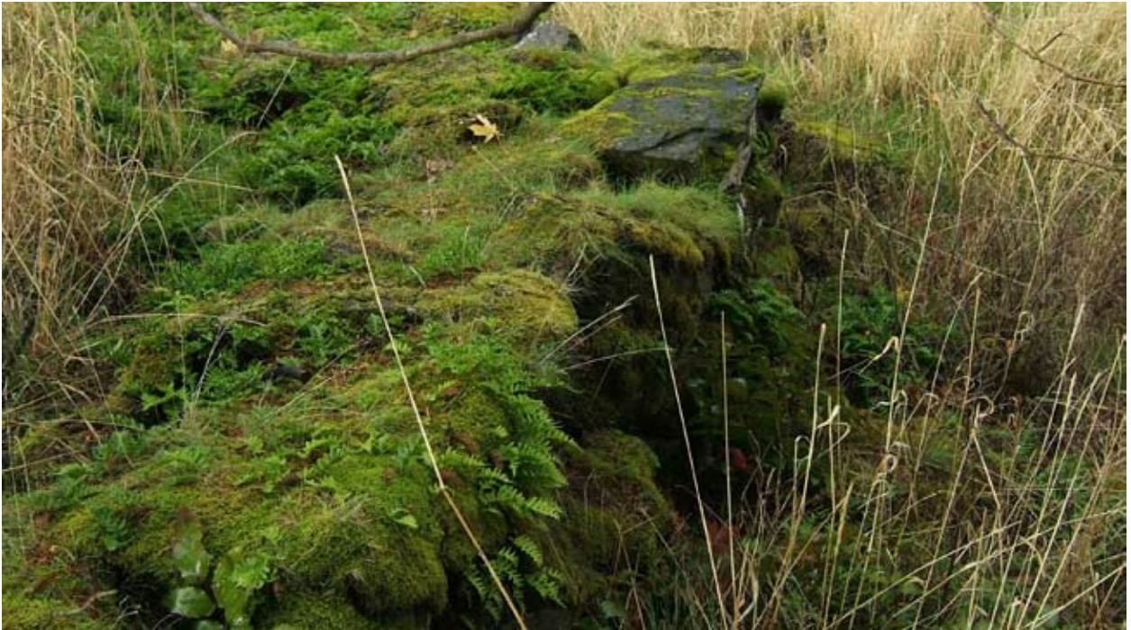
Stonework, drainage area, Ruthton Park
