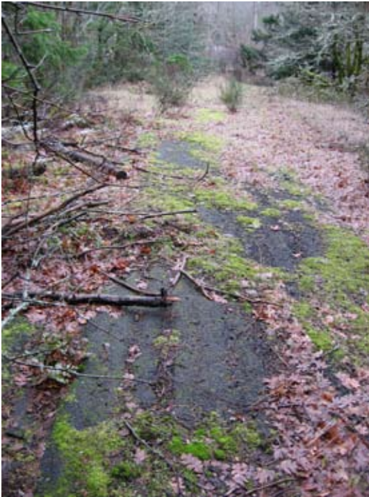
Possible abandoned alignment HCRH.
