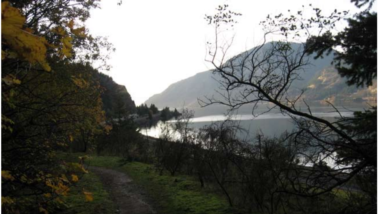
Partially missing pavement, contemporary view, Mitchell Point Segment 2.
