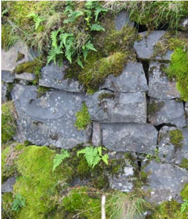
Detail, Cabin Creek retaining wall
