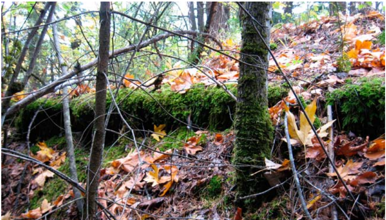
Pavement edge, washout at Mitchell Creek, Mitchell Creek Segment 2
