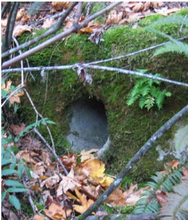
Concrete culvert, concrete head wall, Mitchell Point 2
