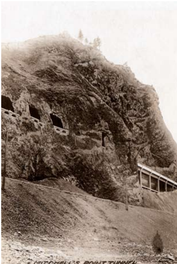
Mitchell Point Tunnel was a precedent for several National Park tunnels, including the Zion - Carmel Tunnel, Zion National Park. Photo courtesy of ODOT.
