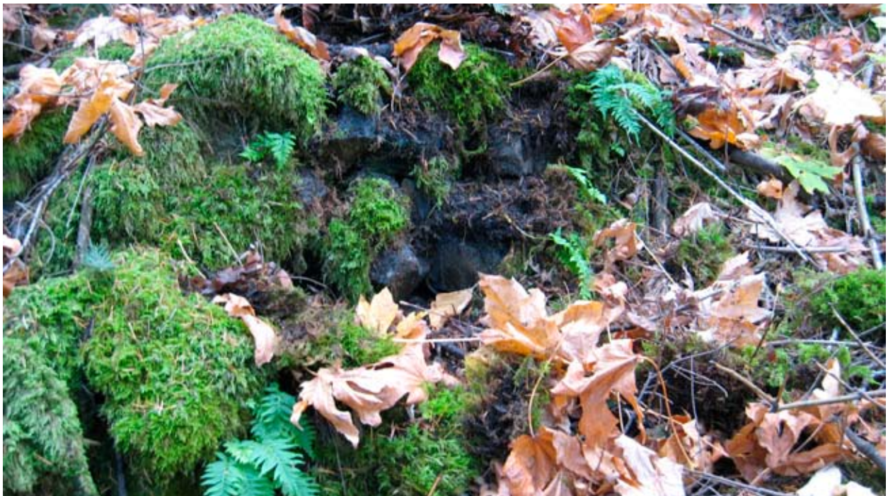
Battered stone retaining wall/ rubble fill. Viento Segment 1.
