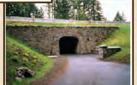
This new undercrossing of Interstate 84 was constructed as part of the Historic Columbia River Highway State Trail Project between Eagle Creek and Cascade Locks.
