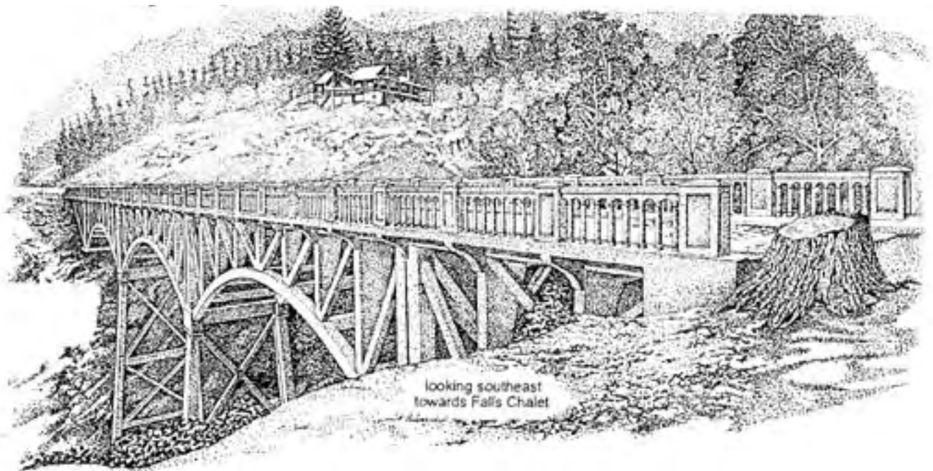
Figure 12—Latourell Bridge looking Southeast towards Falls Chalet
