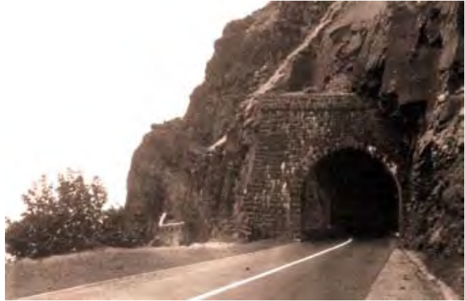
Figure 84—1920s Photo of West Portal of Mosier Twin Tunnels
