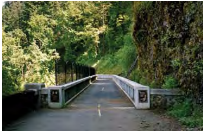
Figure 82—Toothrock Tunnel Bridge
