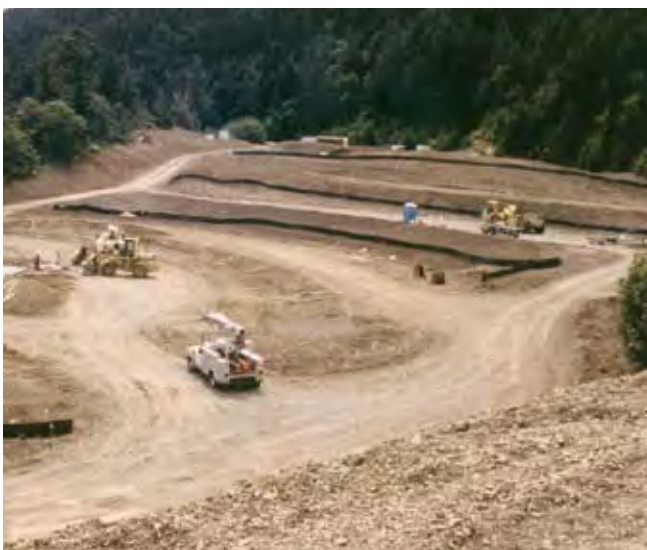
Figure 95—Hanel Quarry Overflow Parking in the Process of Construction
