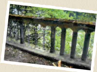
Prior to restoration, the railing in the Toothrock (above) and Ruthton Point (below) Viaducts showed marked deterioration.
