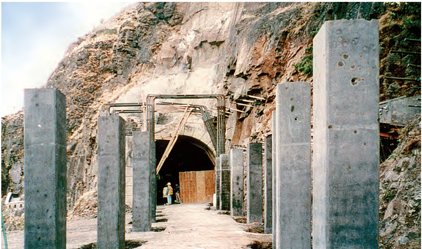
Figure 110—Rockfall Catchment Structure During Construction
