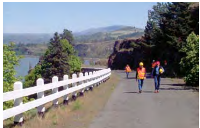
Figure 93—Newly constructed Guardrail
