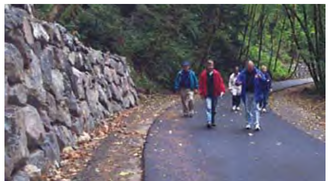
Figure 106—Rockery retaining wall
