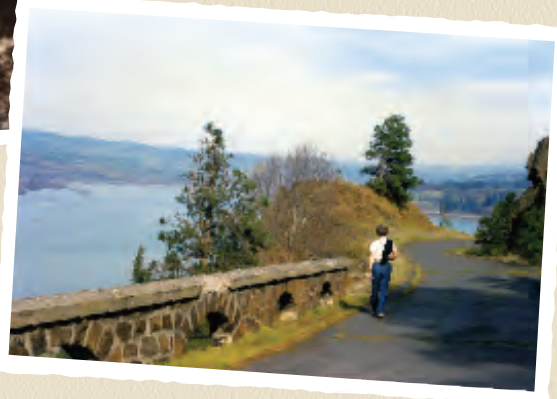
Above and at left: The original highway railings and rubble masonry parapet walls have deteriorated and require restoration. These are photographs of the Ruthton Point area prior to the renovations that have been completed in that section of the State Trail.
