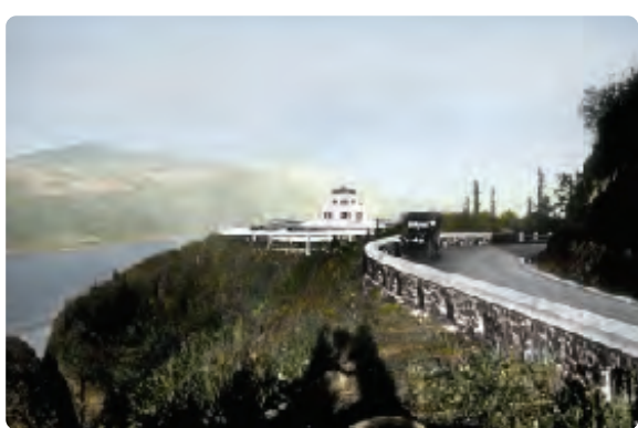
This 1920s hand-painted glass slide was taken looking towards Crown Point and Vista House, with the rubble masonry parapet wall in the foreground. Vista House was constructed beginning in 1916 as an observatory, a "comfort station" (restrooms) and memorial to the Oregon pioneers.
