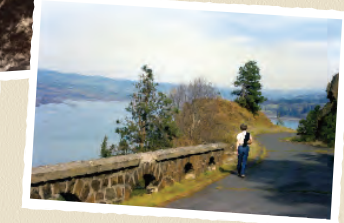
Above and at left: The original highway railings and rubble masonry parapet walls have deteriorated and require restoration. These are photographs of the Rutton Point area prior to the renovations that have been completed in that section of the State Trail.
