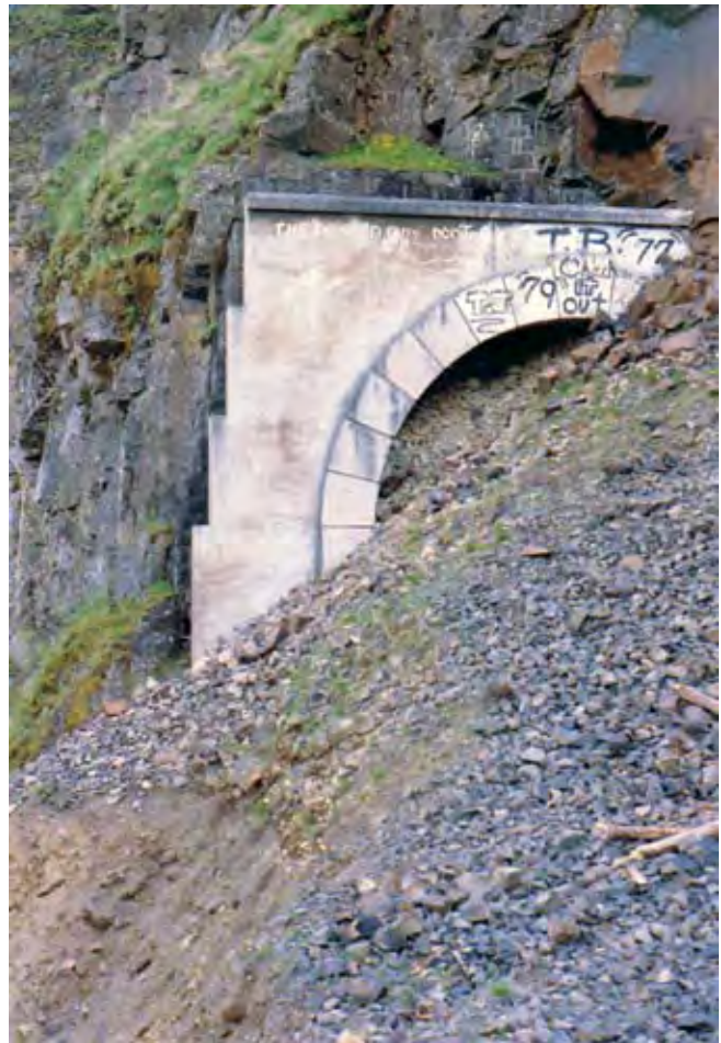
Figure 85—1987 Photo of West Portal of Mosier Twin Tunnels
