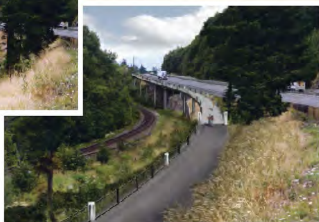
The Warrendale to Moffett Creek State Trail Project would include a lengthy structure to accommodate the steep terrain and limited clearance to the adjoining Union Pacific Railroad. Shown here is a digitally enhanced photograph depicting an artist's interpretation of that proposed structure. Above left is the before photograph of the location of the proposed structure.
