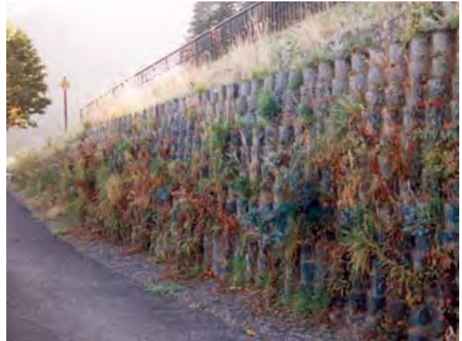
Figure 100—GeoWeb Retaining Wall supports a Wide Variety of Vegetation
