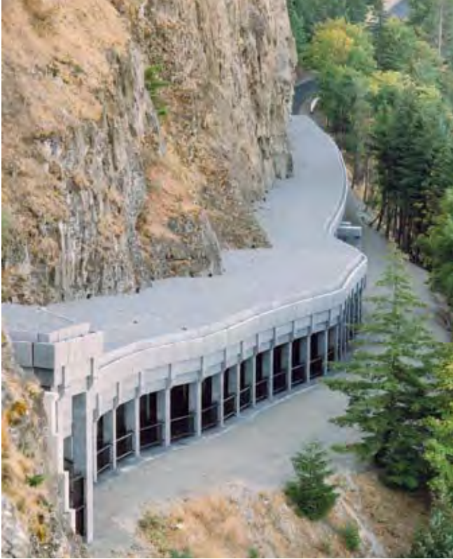
Figure 89—Rockfall Catchment from Above
