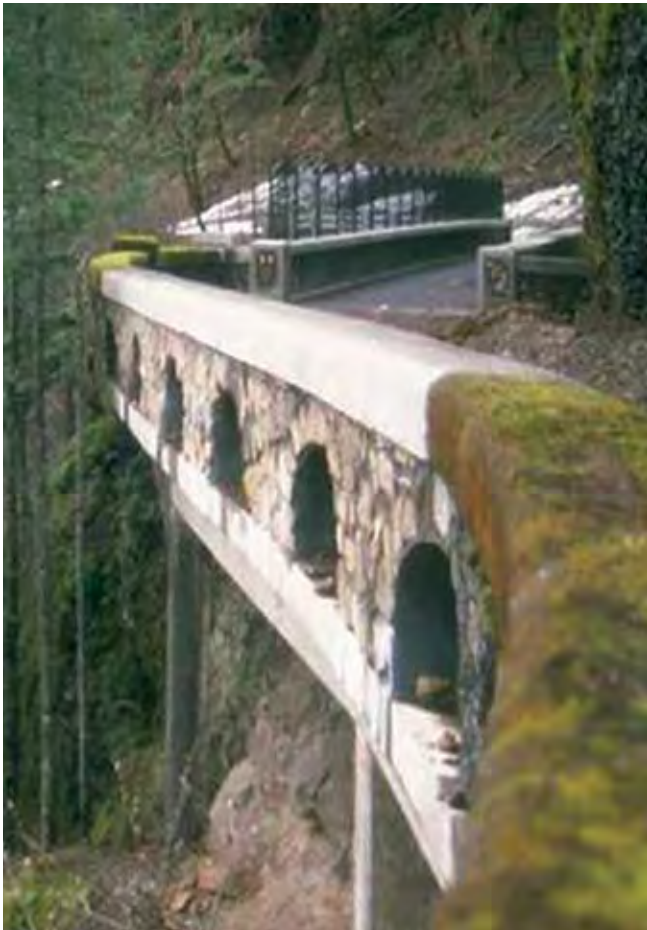
Figure 81—Eagle Creek Viaduct Repaired
