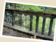
Prior to restoration, the railing in the Toothrock (above) and Rutton Point (below) Viaducts showed marked deterioration.
