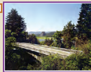
This project also included rehabilitation of the railings on both the Tanner Creek and Moffett Creek bridges (pictured above). Additional interpretive signs and caps for street signs in Cascade Locks and Hood River were also part of the Unit 2 project.
