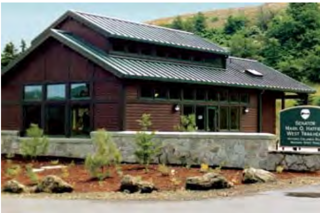
Figure 92—Twin Tunnels Visitor Station
