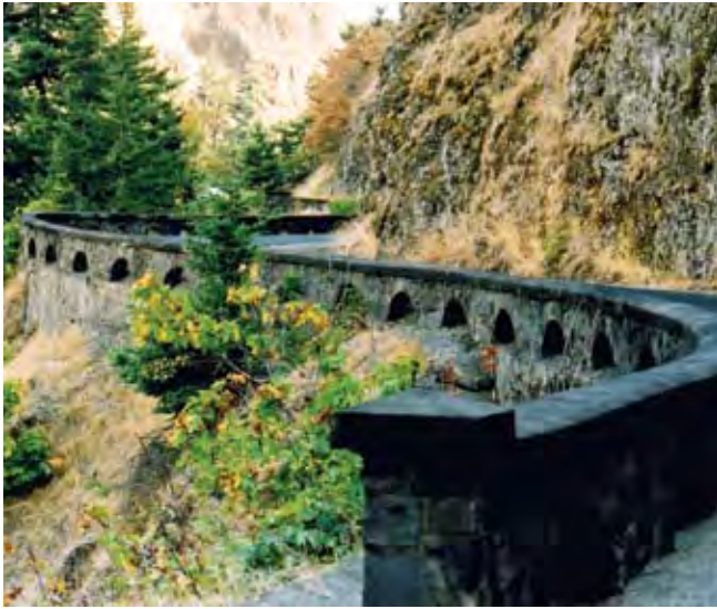
Figure 94—Rock Wall repaired near Inspiration Point
