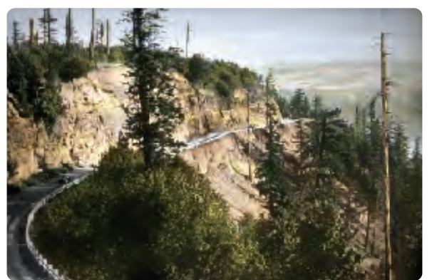
The Historic Columbia River Highway was constructed between 1913 and 1922 with maximum 5% grades and two-rail wooden guardrail that became a national standard for guardrail.
