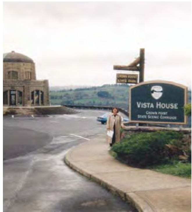
Figure 67—The Thematic Site Sign at Vista House used the existing Stone Base and the Thematic Sign Shape and Colors
