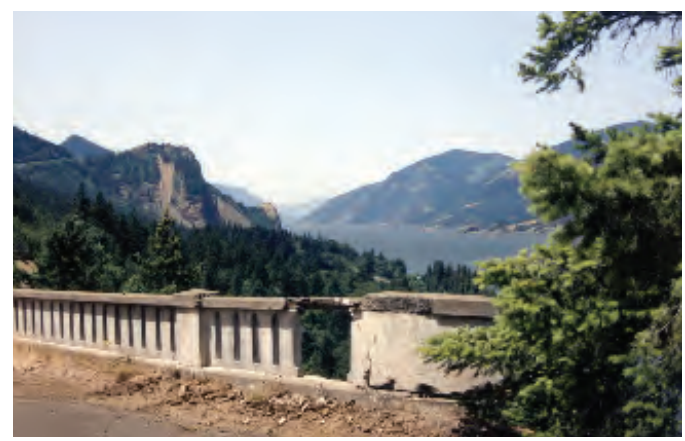
Prior to restoration, the railing in the Toothrock (above) and Ruthton Point (below) Viaducts showed marked deterioration.
