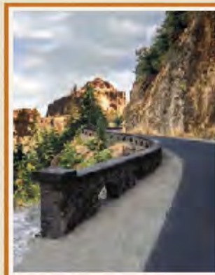
Picture left: Newly constructed rubble masonry parapet rock wall at Bingen Overlook.
