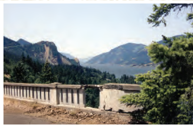
Prior to restoration, the railing in the Toothrock (above) and Rutton Point (below) Viaducts showed marked deterioration.
