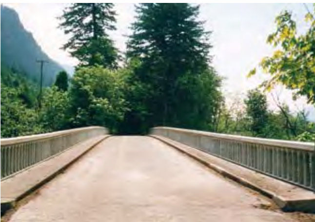
Figure 103—Moffett Creek Bridge railing was replaced to match the original
