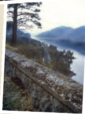
Above and at left: The original highway railings and rubble masonry parapet walls have deteriorated and require restoration. These are photographs of the Ruthton Point area prior to the renovations that have been completed in that section of the State Trail.
