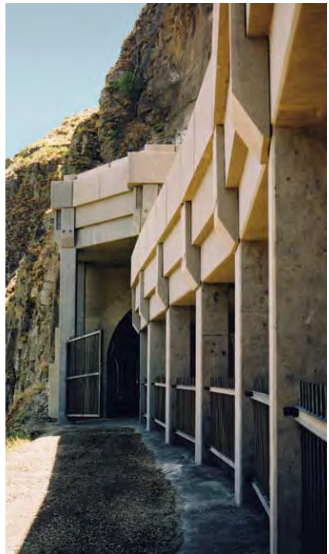
Figure 88—Rockfall Catchment
