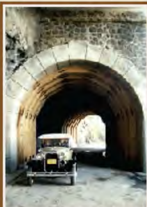
Phase one of the Hood River to Mosier Project included reopening the Mosier Twin Tunnels.
