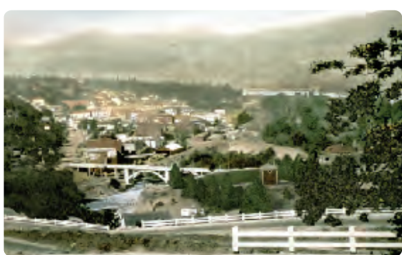
Just east of the city of Hood River, the Hood River Bridge was the longest bridge on the highway, leading to the Hood River Loops. The bridge was demolished in 1982.
