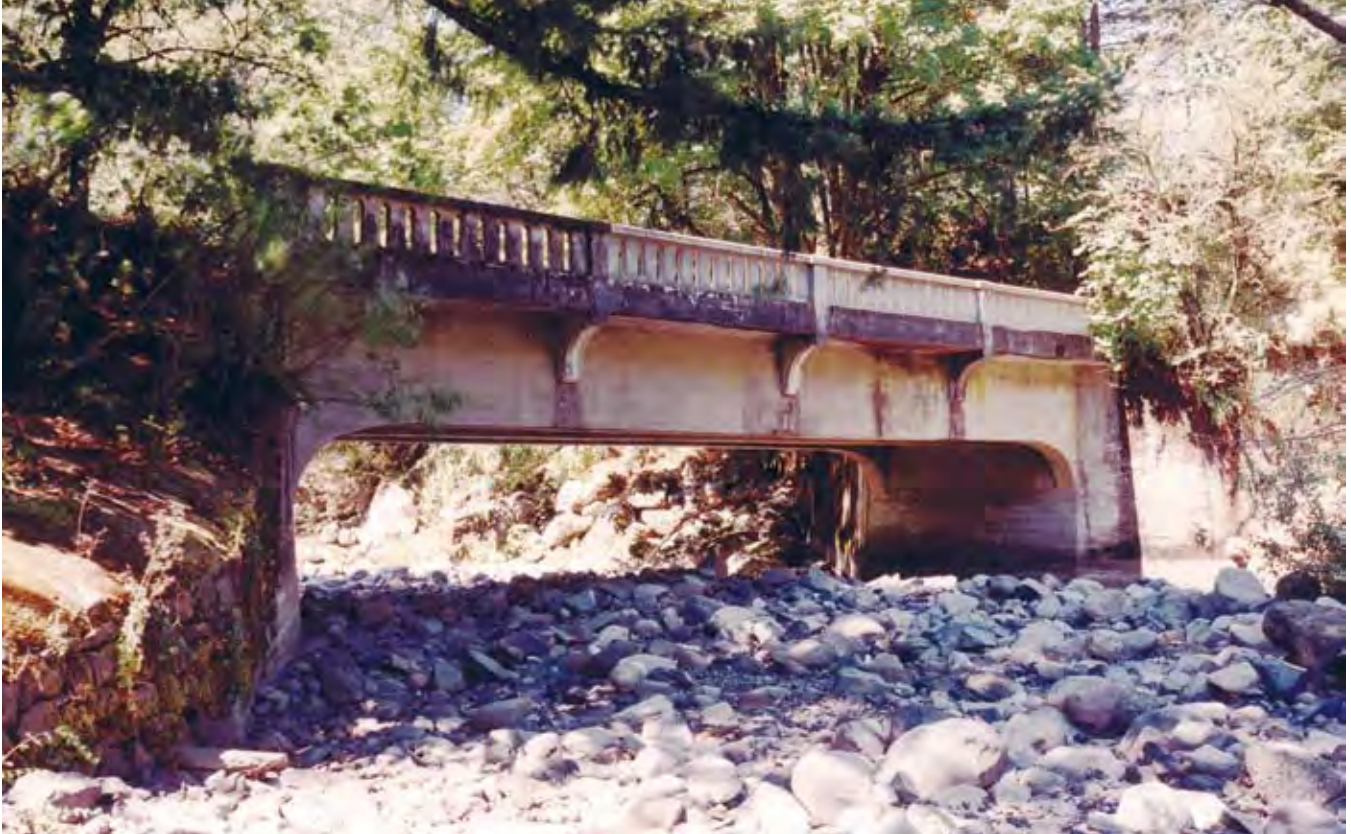
Figure 102—Tanner Creek Bridge Railing Repaired
