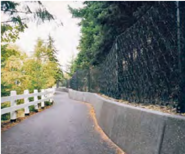
Figure 107—Rockfall Mitigation between Starvation Creek and Viento
