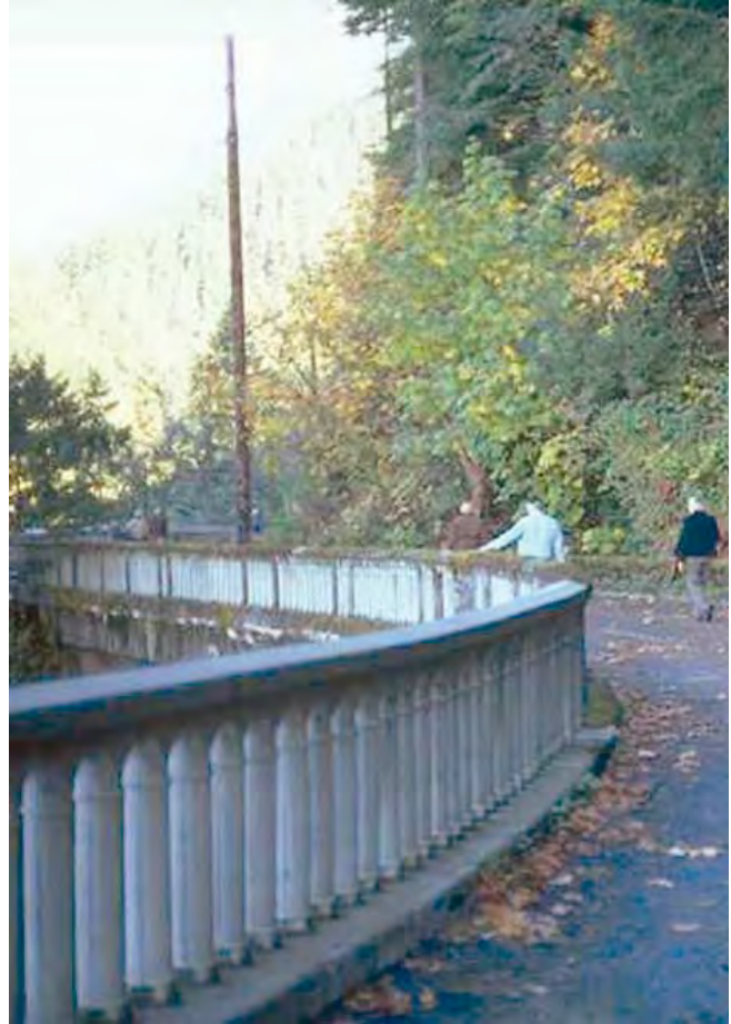
Figure 78—Toothrock Viaduct Railing Repaired
