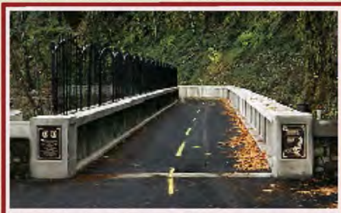
A new bridge, the Toothrock Tunnel Bridge, was required over the east portal of the Toothrock Tunnel. This project won an award for the best non-highway bridge.
