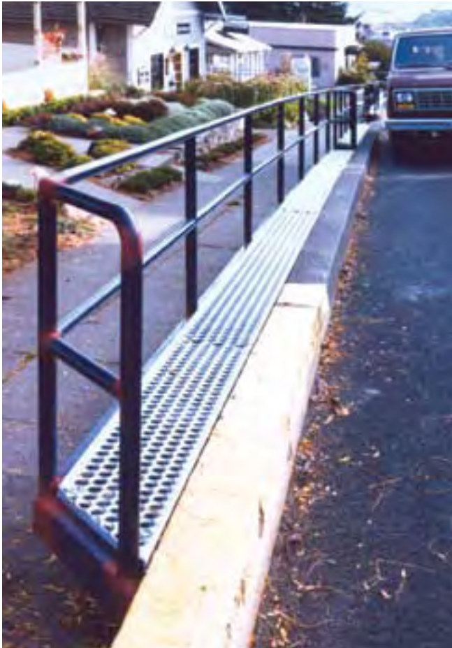
Figure 31—Pedestrian Railing in Hood River
