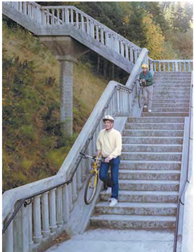
Figure 83—Groove included on Stairway allows for Bike Access
