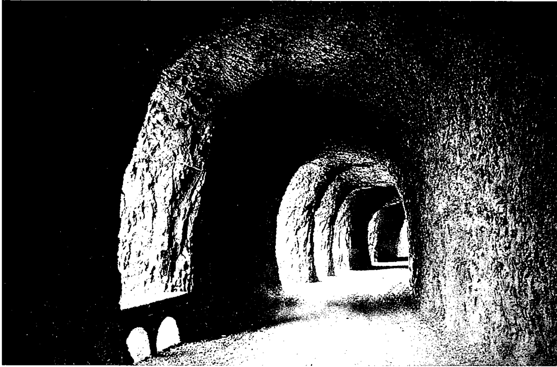
Figure 16 Mitchell Point Tunnel - the Tunnel of Many Vistas
