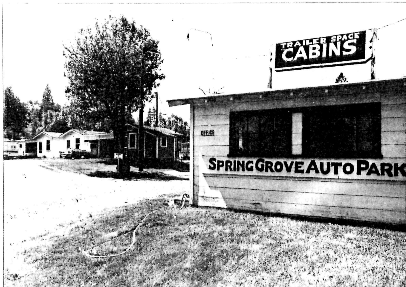
Spring Grove Auto Park on Cascade Street, Hood River. Tent campers probably gathered around the natural spring on this site before the cabins were built in 1925. It is now a mobile home park. [Mile 52.3]
