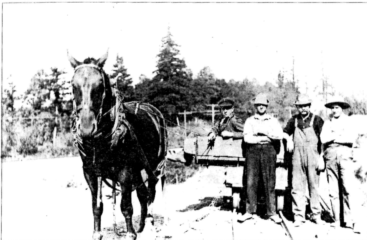
Fred Luscher (in wagon) and friends helping to build the Columbia River Highway. (OHS #62699)
